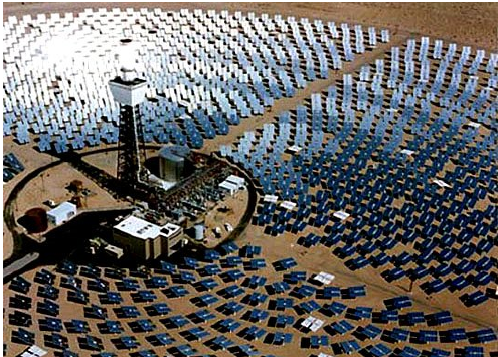
World Largest Solar Power Station in Germany
