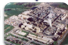
Pilot plant 200 bbl/day Australia
